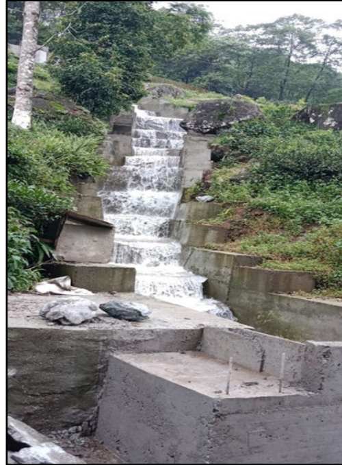
(Extension of Forebay spillway at MungpooKalikhola Hydel Power)
