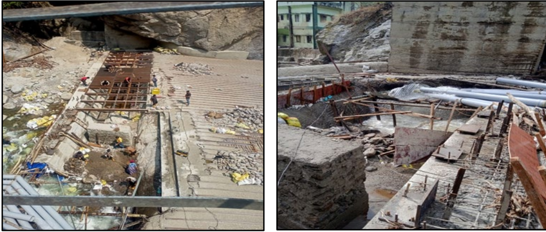
(Repairing work going on at Diversion Structure & Trash Rack)
